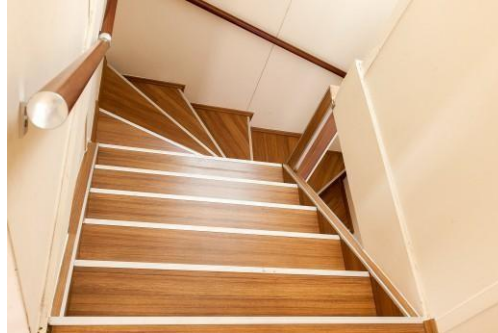
Stairs with timber cover
